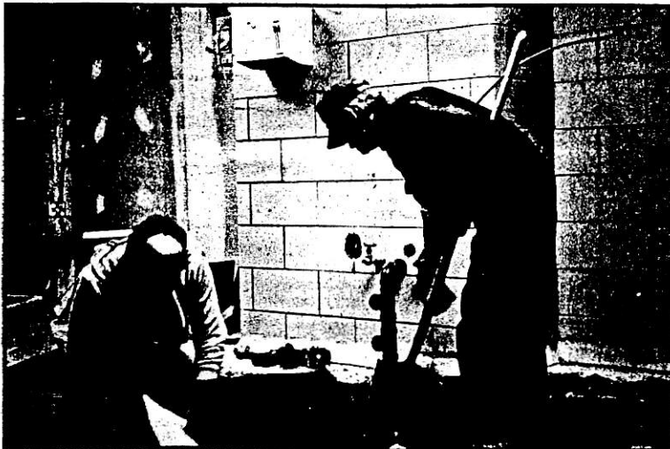
The canteen and parts of the cafeteria's cooking area underwent a $7,000 repair project during the semester break. Here, Physical Plant employees work on cafeteria plumbing.
